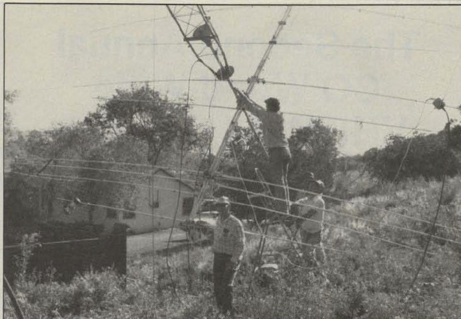
I have a Rohn Model 45 crank-over, and it proved to be no easy job getting the beam on mast—in the upside-down position. However, with the help of some intrepid local amateurs, we got the job done.
