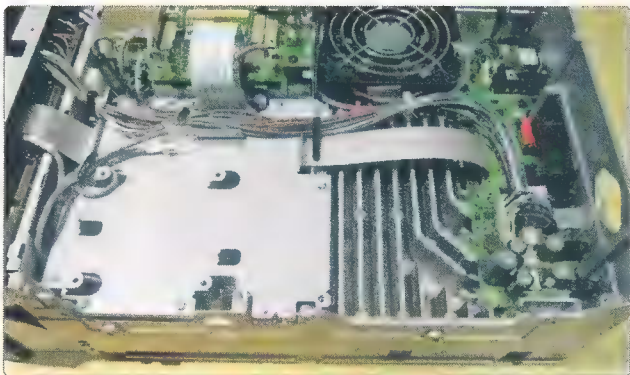
The location for the installation of the UX-9100.
