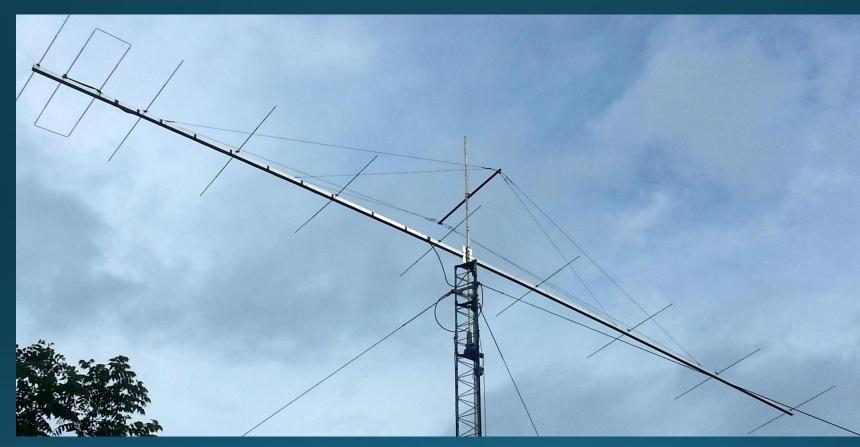
Nice upper double boom truss: Cross bar is high enough and wide enough to create good pulling geometry. Intermediate boom guys provide additional tweaking of boom straightness.
