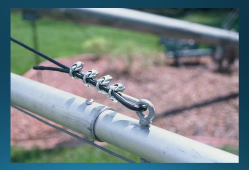
Doing the boom truss end the right way:
