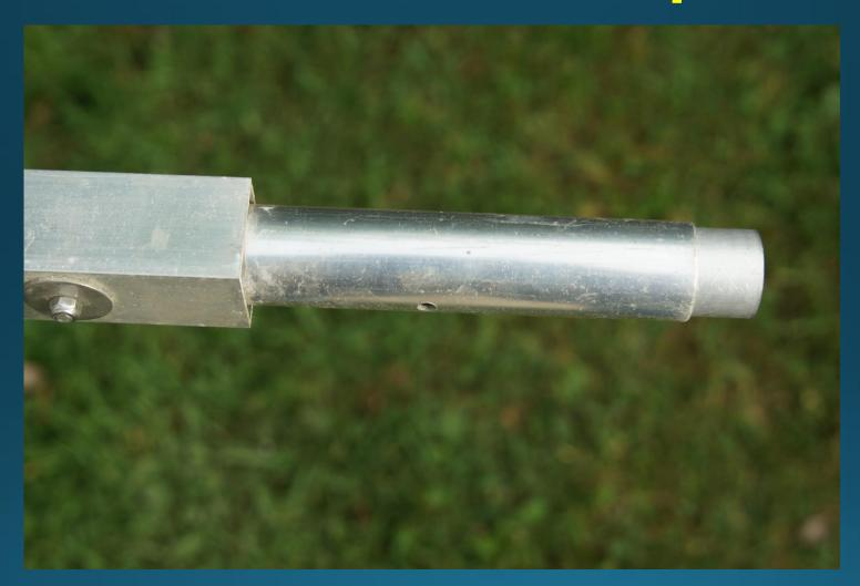
Round splice tube may be reinforced via inner sleeve(s).
