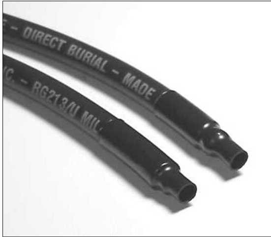
Figure 20. After shrink wrapping.
