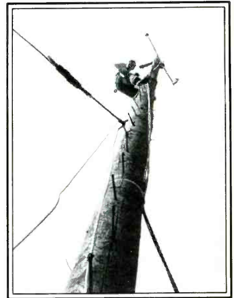
A Skytrooper of the 3rd Brigade, 1st Cavalry Division, installed an antenna for a tactical operations center in Bien Hoa, Republic of Vietnam. (U.S. Army photo by SP4 Larry Buehner, Army News Features.)
