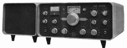
The KW2000E transceiver incorporates a number of improvements over previous models the most important being, improved cross modulation performance, a 500 KHz VFO with greater stability and full amateur band coverage from 1.8 MHz to 30 MHz as standard.
