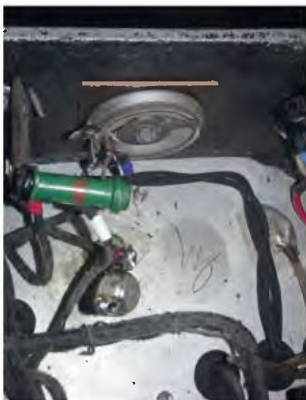
The old carrier meter zero adjustment is shown above with its replacement circuit at right ( 200\Omega potentiometer R10).
